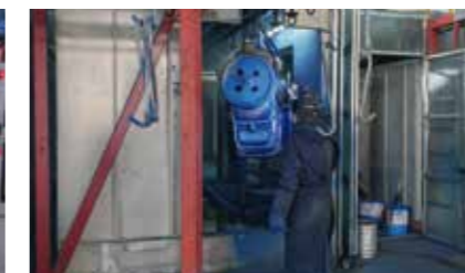
Valve Spray Coating
